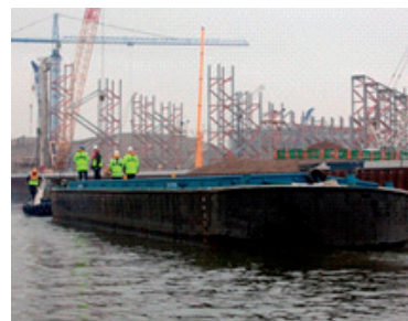
An early delivery by water facilitated by the Aquatics Centre contractor
