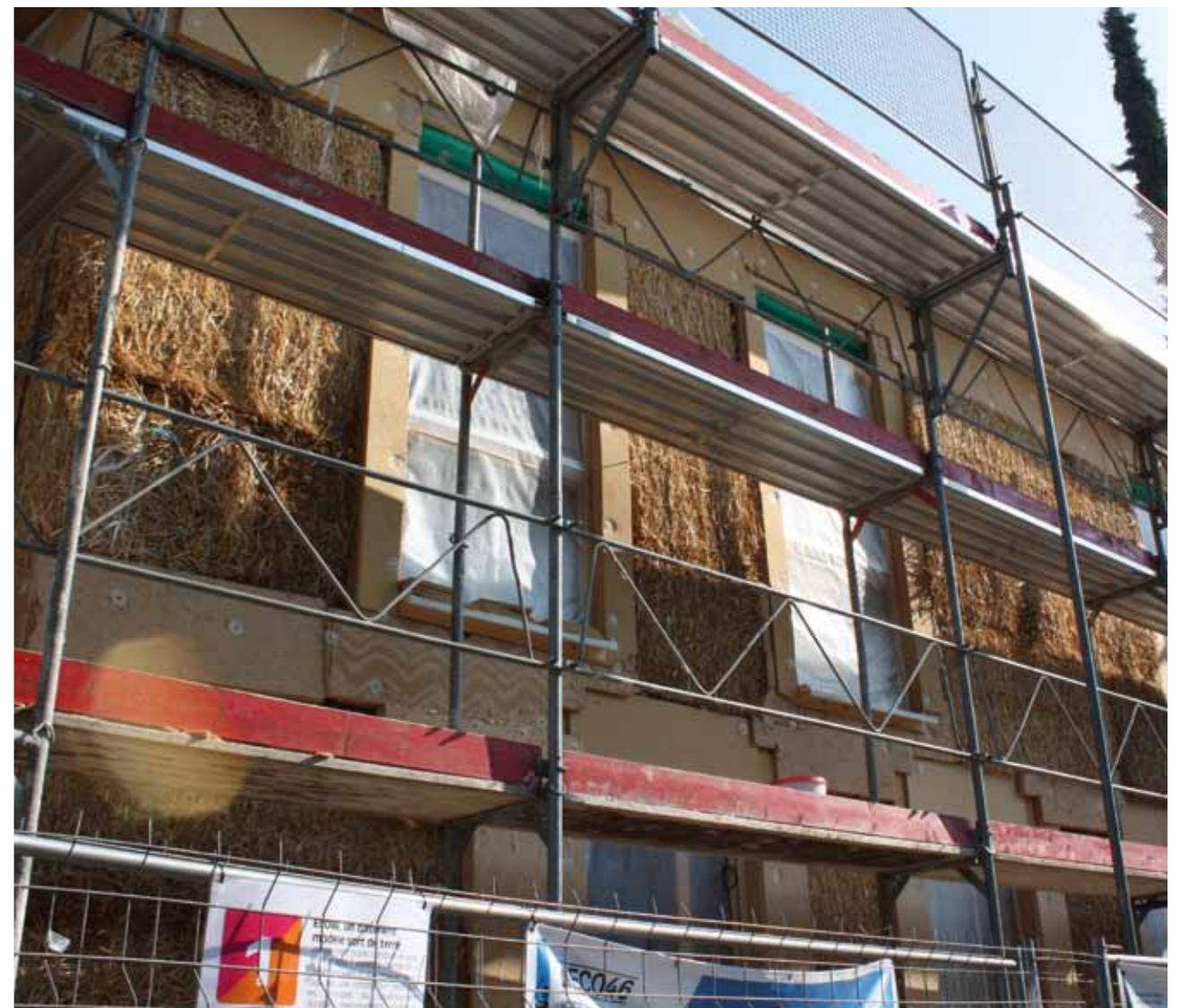
Compressed straw has been proven to be an efficient, naturally-sourced building material and insulator. © M. Barra
