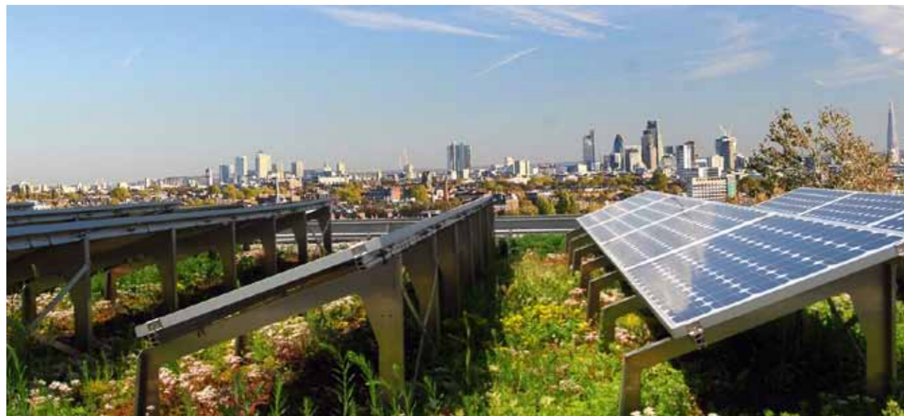
Combining solar energy and plant life brings mutual benefits: the vegetation cools the panels and increases their productivity, while they provide shade and habitat diversity for surrounding flora. © 2015 Green Roofers Ltd
