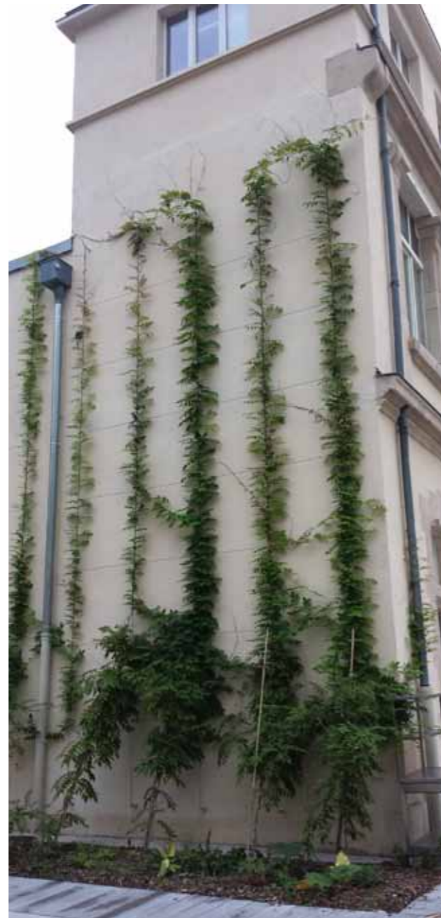
Walls without windows and gable walls can host climbing plants, which protect the building against extreme weather, cooling the air and providing a habitat for small animals. © M. Barra
