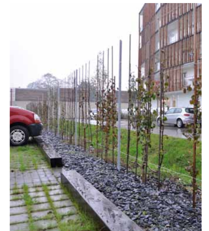
Car parks, pathways, and fire access areas are all spaces that can be developed without the use of impervious surfaces. © G. Lecuir
