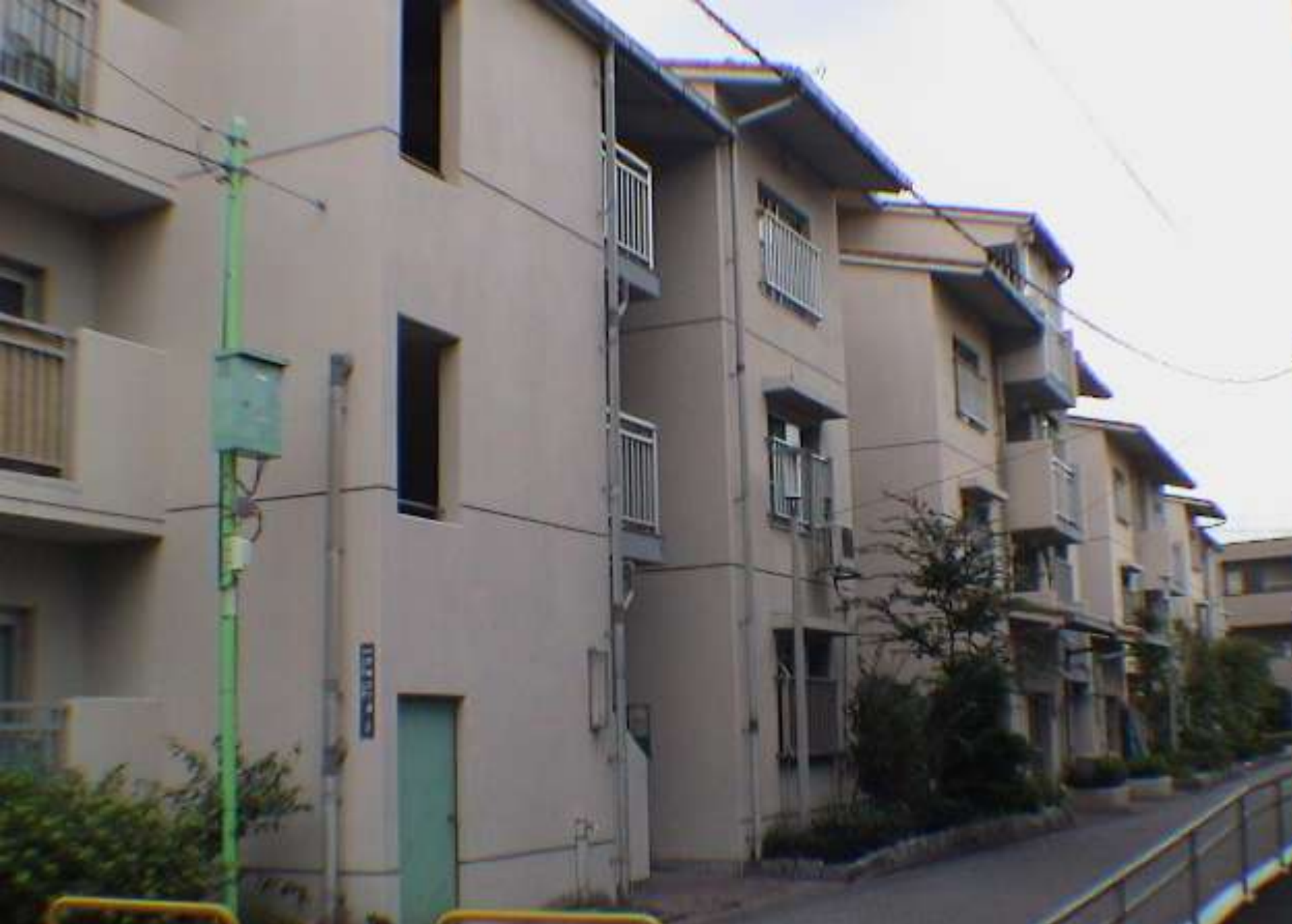
Example of middle rise scale housing ( Public housing at Sumida ward)
