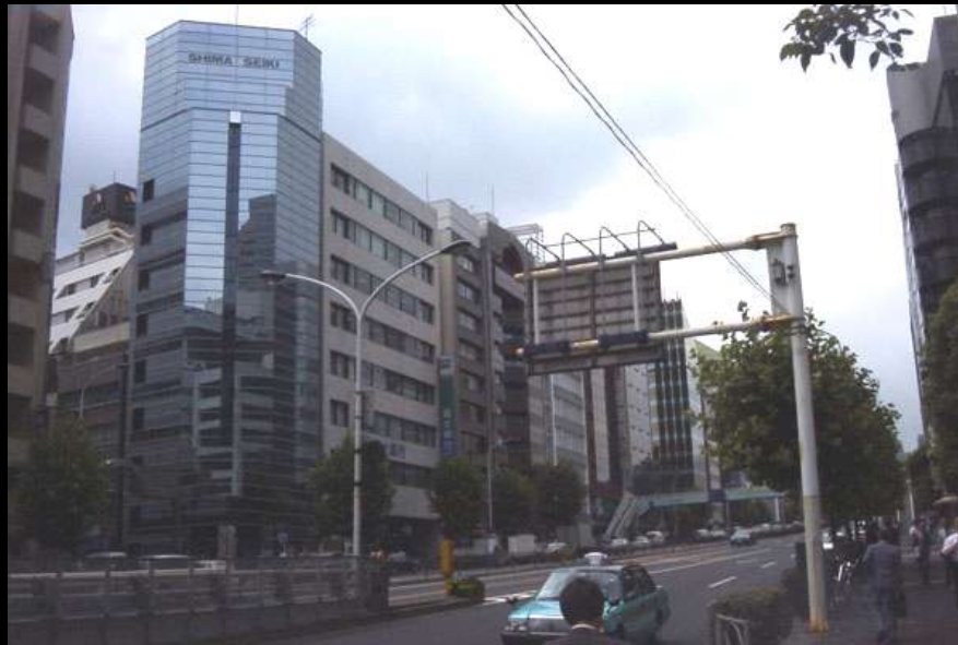
Penthouse (Machine Room)
