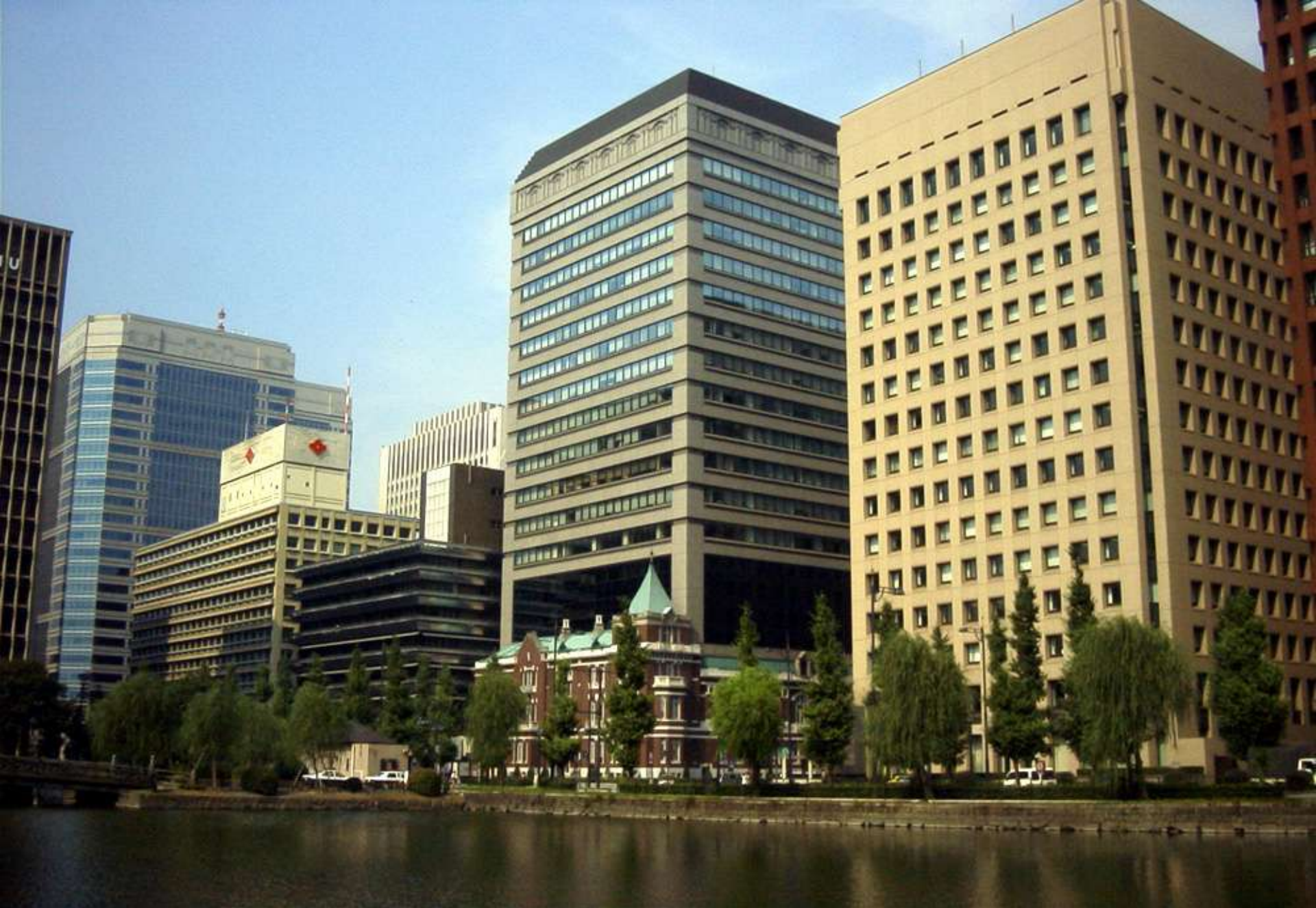
Large buildings along the wide streets around the block(Marunouchi)
