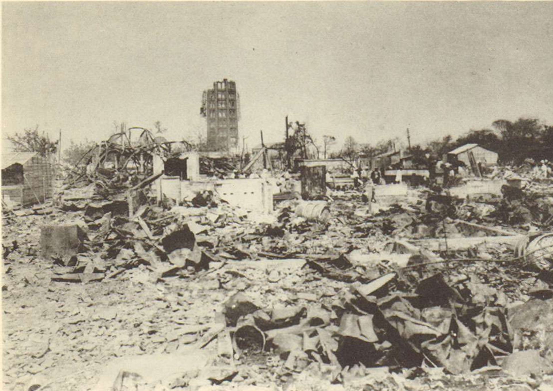
Asakusa district after the Great Kanto Earthquake(1923)
